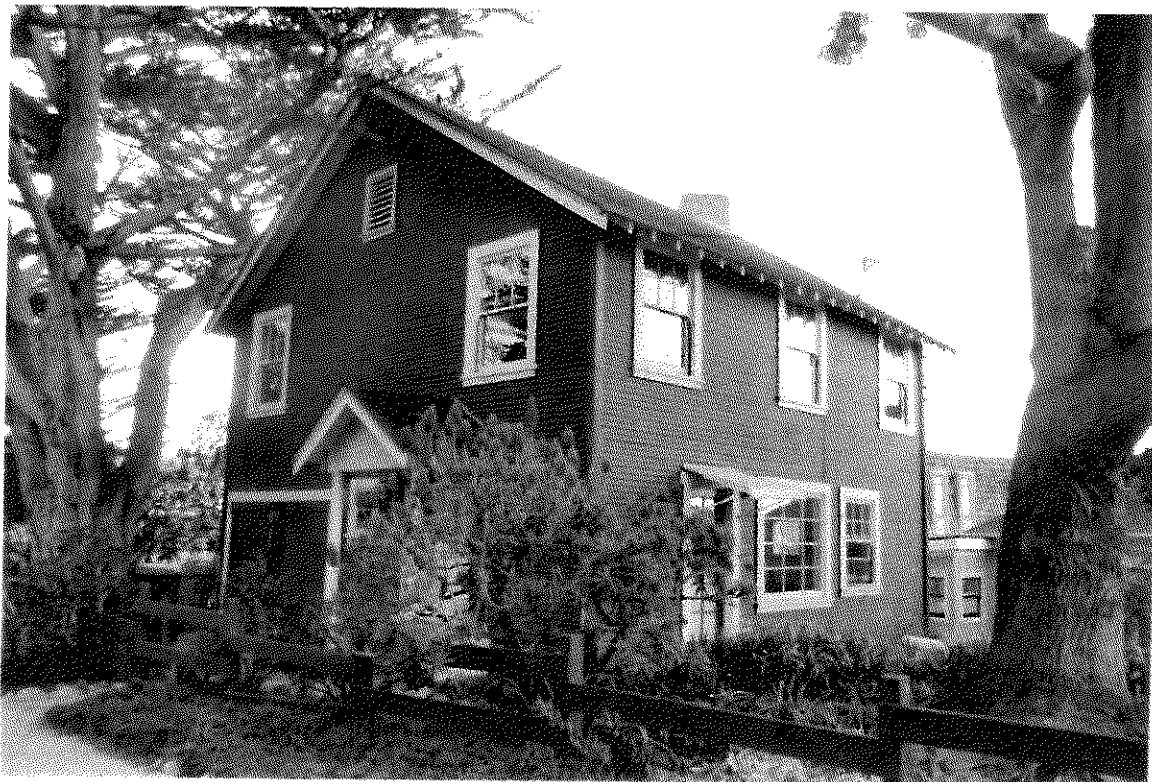
Photo #2. Looking NW at the south facing facade & east side-elevation, October, 2014.
