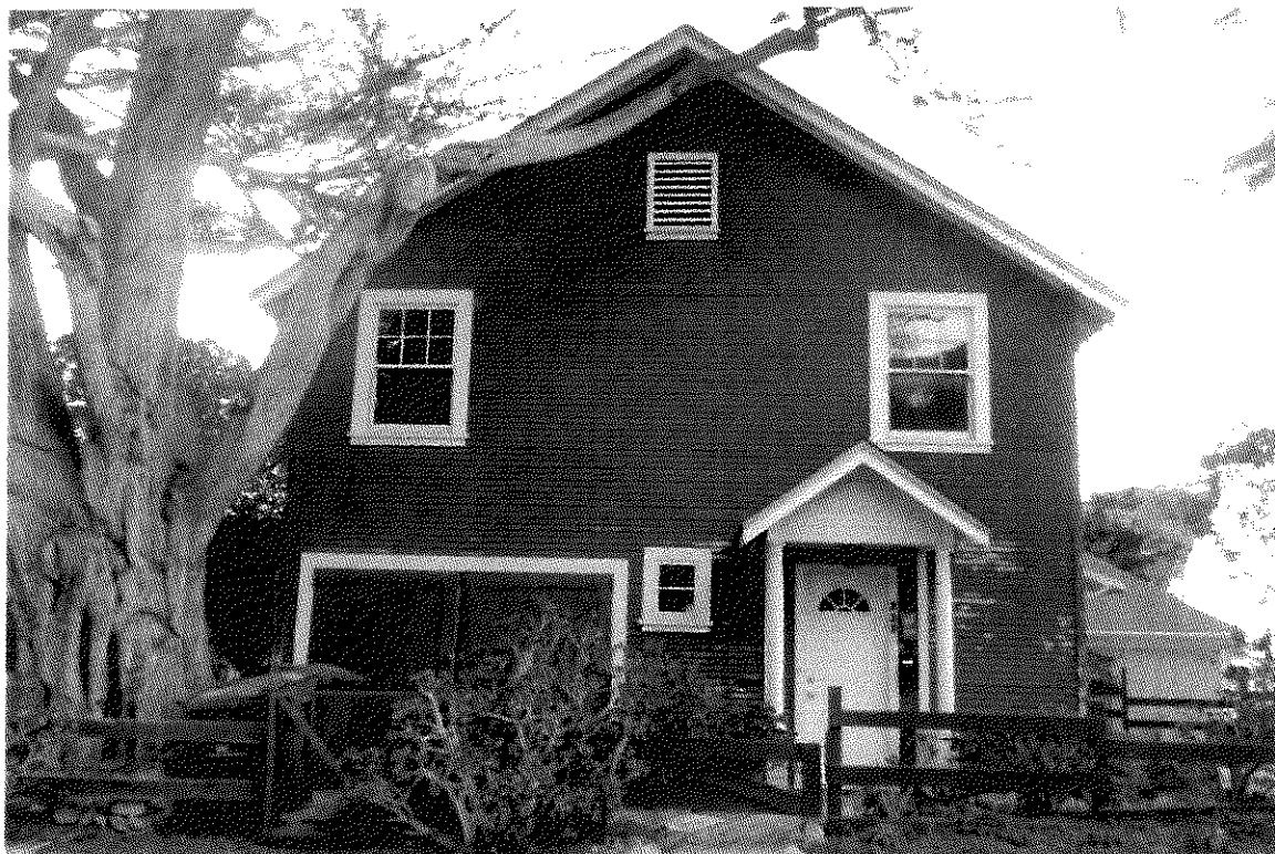
Photo #1. Looking north at the south facing facade, October, 2014.
